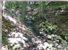
Fig. 6 Boulder armoring failure and underlying blanket mobilization in a ravine tributary just south of the Calder Art Center. Photo taken by T. LaCross, 08/01/06.
