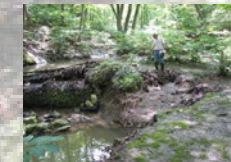
Fig. 7 Lowest check dam in the Little Mac ravine showing increased erosion due to the stream bypassing it during high flow conditions. Photo taken by P. Womble, 07/20/06.
