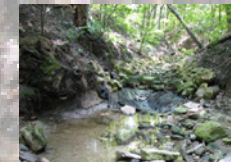
Fig. 8b Boulder armoring failure in Little Mac ravine. Photo taken by P. Womble, 07/20/06.
