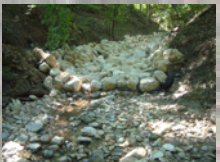
Fig. 8a Boulder armoring newly installed in the Little Mac ravine. Photo taken by P. Videtich, 09/03/02.
